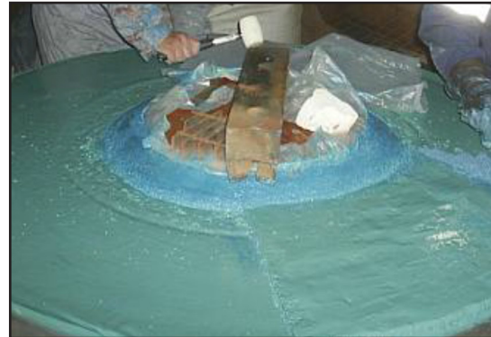
Applying ARC MX1 over primer coat of ARC S2
